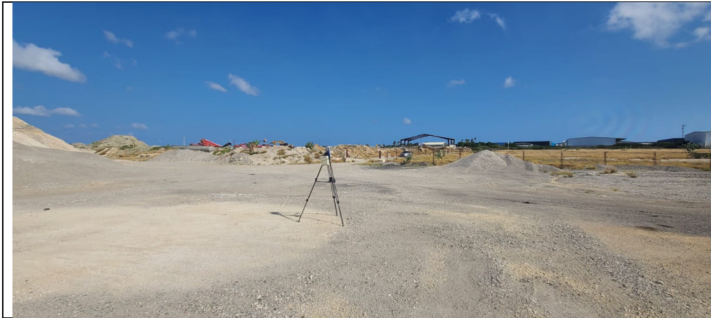
South end of the main road, facing North. Project site is located on the left of the road.
