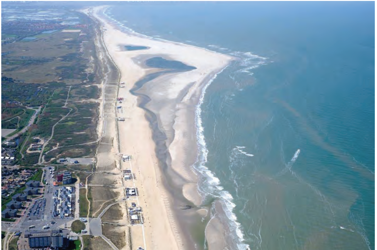
Figure 4.18 Sand Motor seen from the north, 21 July 2015. Courtesy Joop van Houdt/RWS
