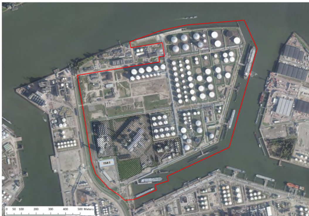
Figuur 4.8: Ligging Tank Truck Loading Rack 2
