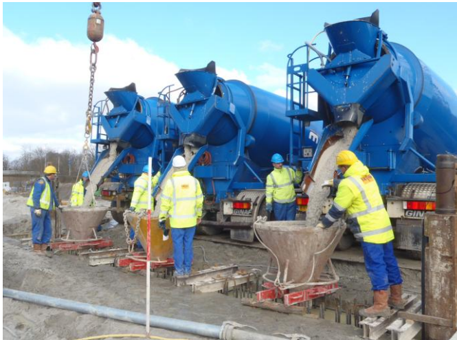
Beton storten in de diepwandsleuf
