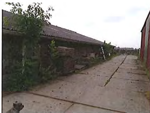
Foto 1: te slopen stal (600 m2)
