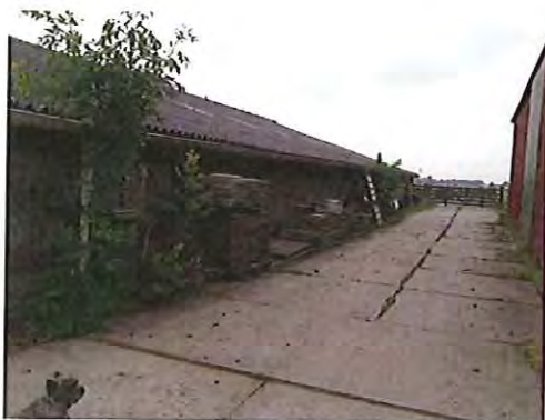
Foto 1: te slopen stal (600 m2)
