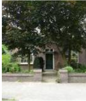
Woning langs Griftdijk
