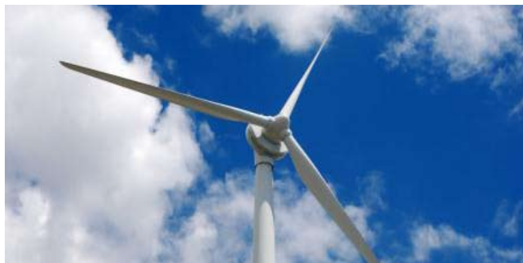
Windenergie langs A50
