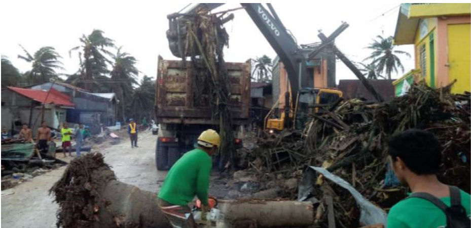
Samar Road facilitates emergency response after Typhoon Haiyan
