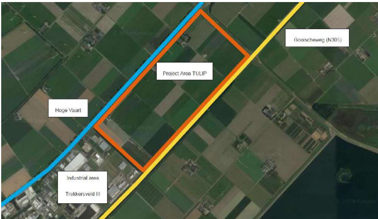
Figure 1: Location of the project area with a satellite image of the current situation.
