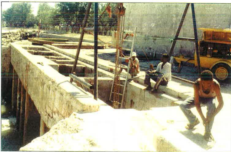
Figure 3.4 – Wave barrier wells at the Palmeiras desaquadouro
