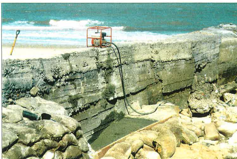
Figure 3.7 – Placing the mass concrete shoulder on the downdrift side of Groyne 33 (photo by Luis Renne)
