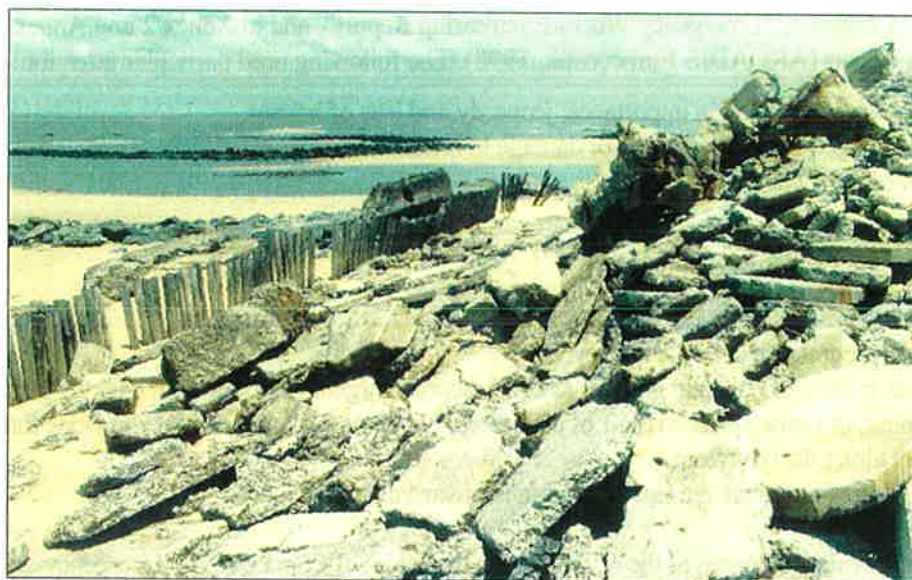
Figure 2.8 – The embattled headland at Punta Gea with rubble defence
