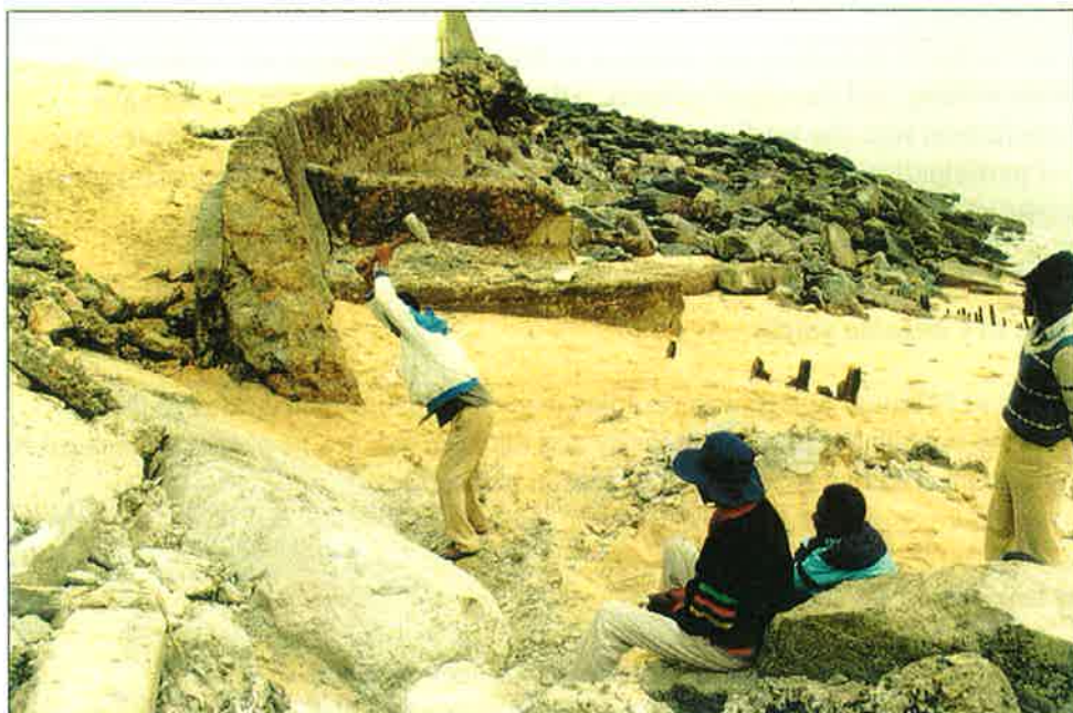
Figure 3.12 – Demolition work at Groyne 4 and adjoining seawall in Ponta Gêa by the Conselho Municipal's Road Brigade
