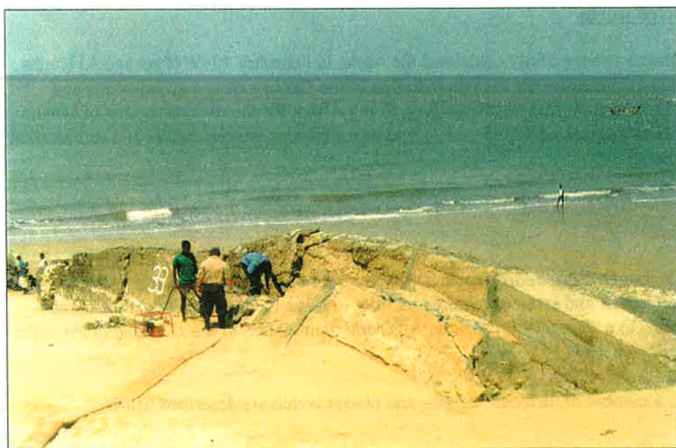
Figure 3.2 – Repair work to Groyne 33 being examined by Project Engineer
