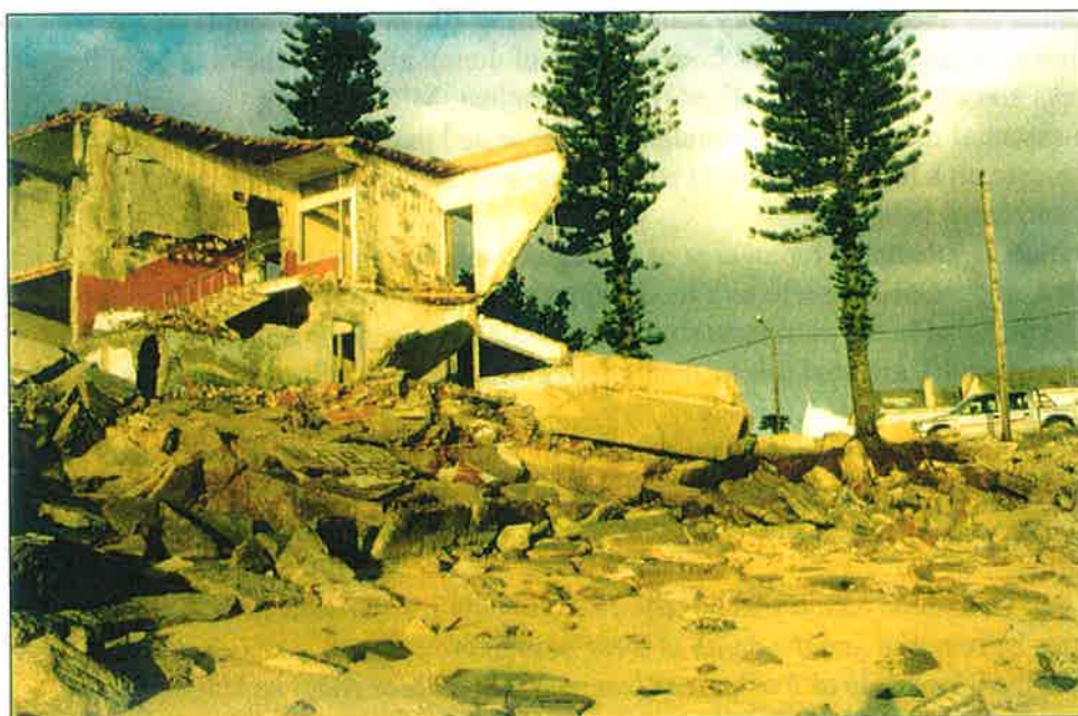
Figure 2.23 - House collapsed into sea at Punta Gea from erosion
