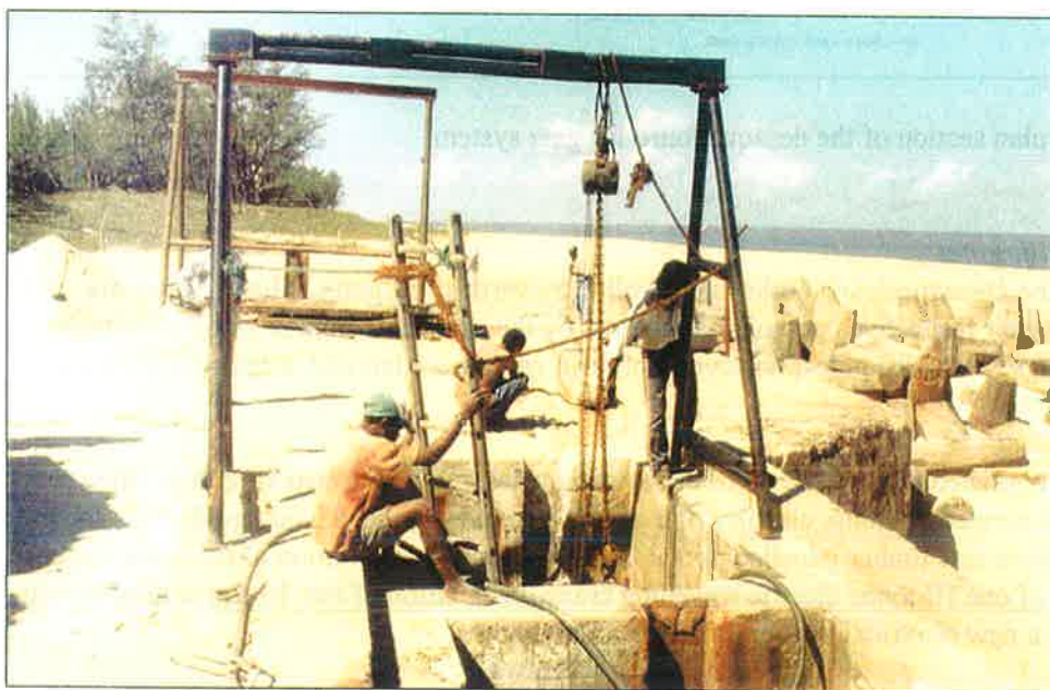
Figure 3.5 – Hughs construction crew removing old stoplogs from the Palmeiras desaquadouro
