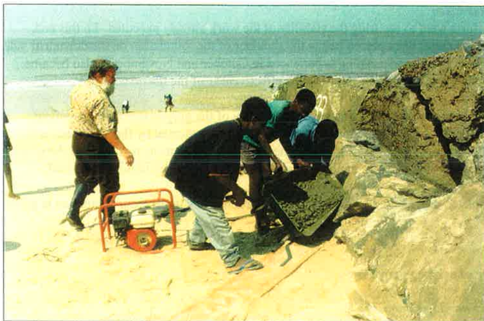
Figure 3.8 – Groyne repair involved considerable hand labor – the Project Engineer inspects work of the Rumdel construction crew
