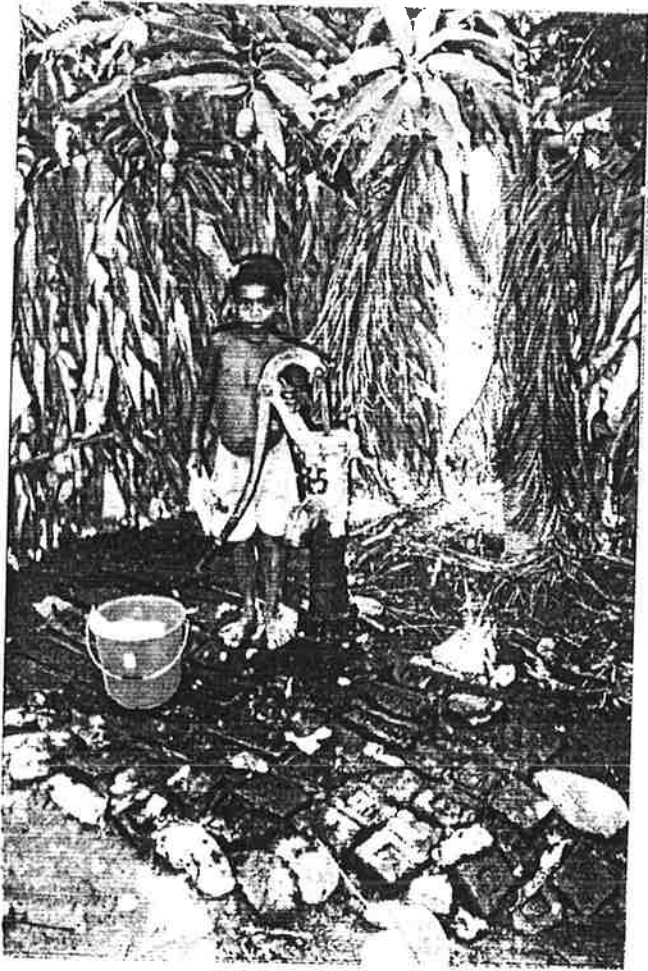
FIG 1 : HTW with dilapidated platform.
