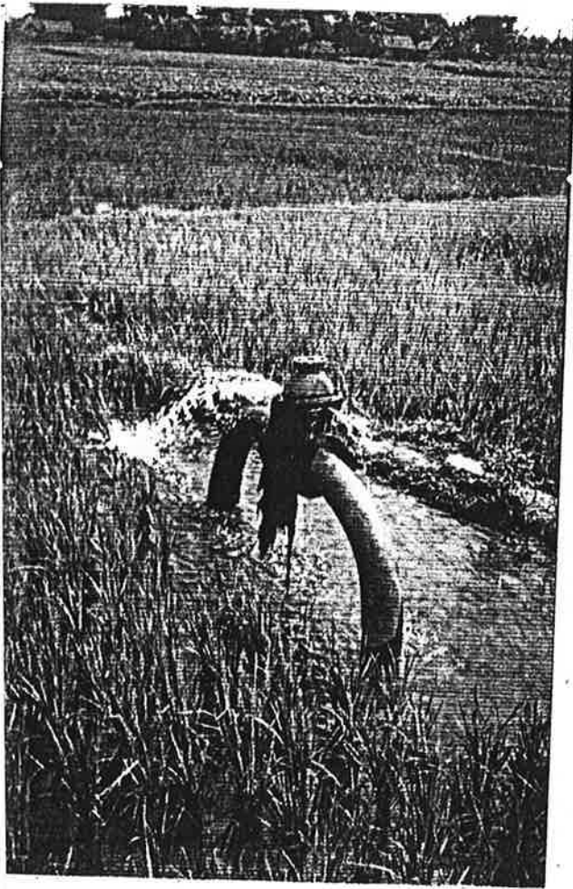
FIG 4(i): Leaking valve forming water pool.
